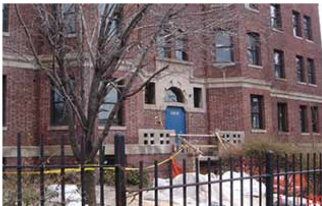
Private renovation: New Jersey Ave at New York Ave
