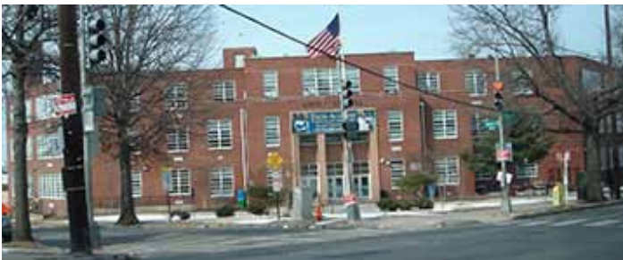
Excel Academy under expansion
