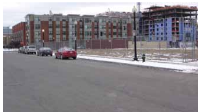
2 M Street under construction
